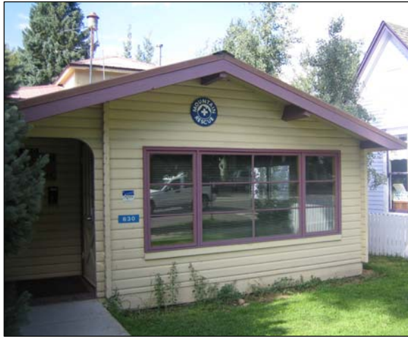
Figure 3. Recessed entrance at 630 Main Street, built in 1965.
