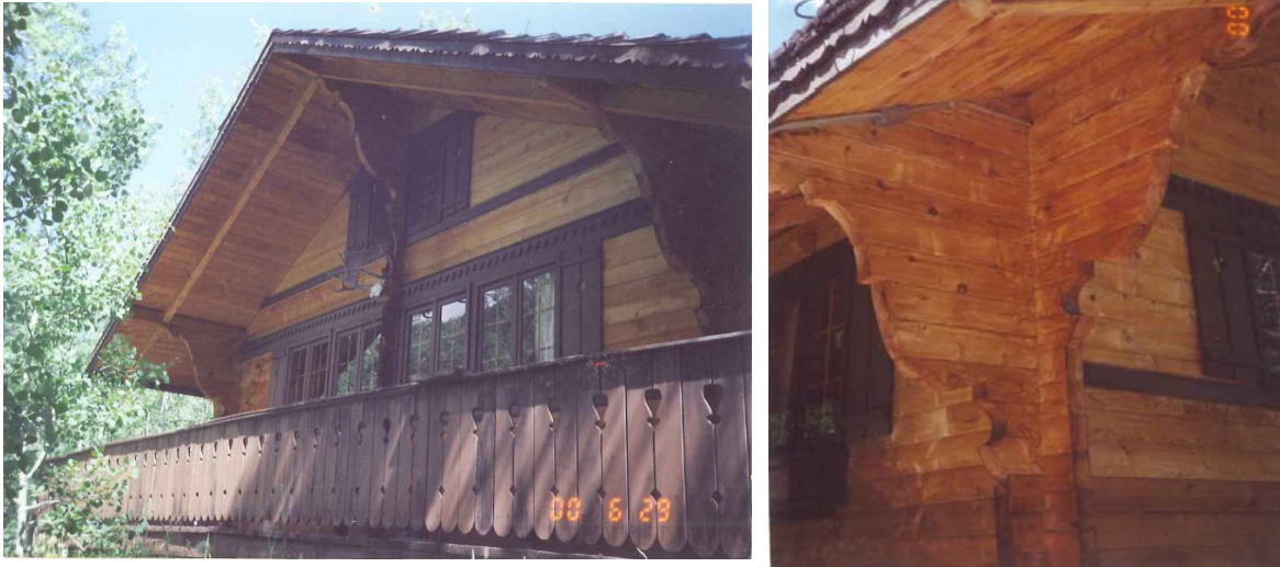
Figure 5. A Chalet Style Pan Abode (demolished)
