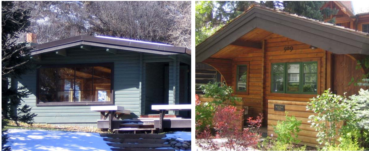
Figure 6. The picture windows of Pan Abodes, as seen at 509 West Main Street, left, and 1355 Sage Court, right.
