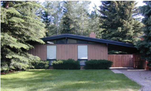
Figure 48: 625 Gillespie Avenue, designed by Benedict. City of Aspen files.
