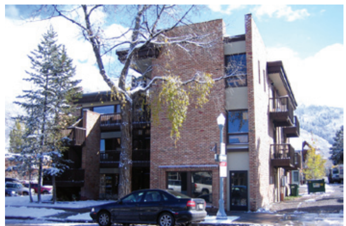
Figure 42: 300 South Spring Street, designed by Heneghan and Gale. City of Aspen files.
