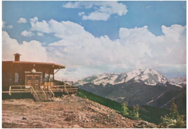
Figure 13: Sundeck atop Aspen Mountain, designed by Benedict. Courtesy AHS.
