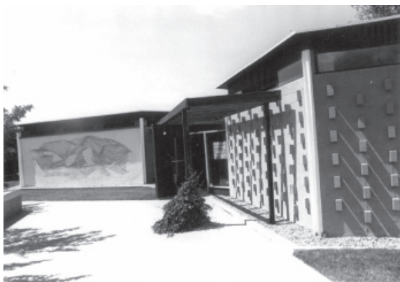
Figure 36: Koch Seminar Building, designed by Bayer. City of Aspen files.
