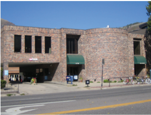
Figure 16: National Bank of Aspen, now US Bank, designed by Caudill. City of Aspen files.
