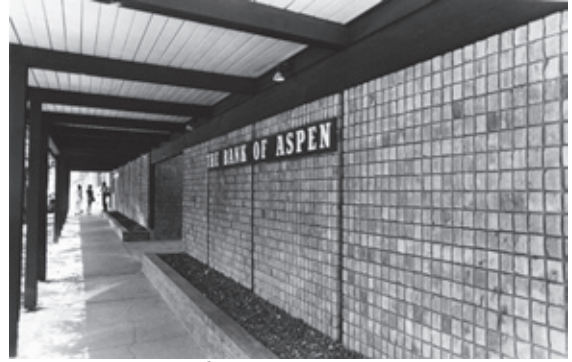
Figure 15: Bank of Aspen, now Wells Fargo Bank, designed by Benedict. Courtesy AHS.
