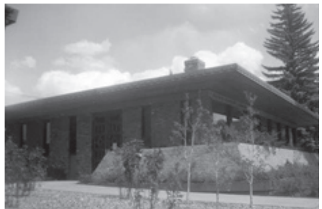
Figure 44: 120 East Main Street, originally the Pitkin County Library, designed by Bayer and Benedict. City of Aspen files.
