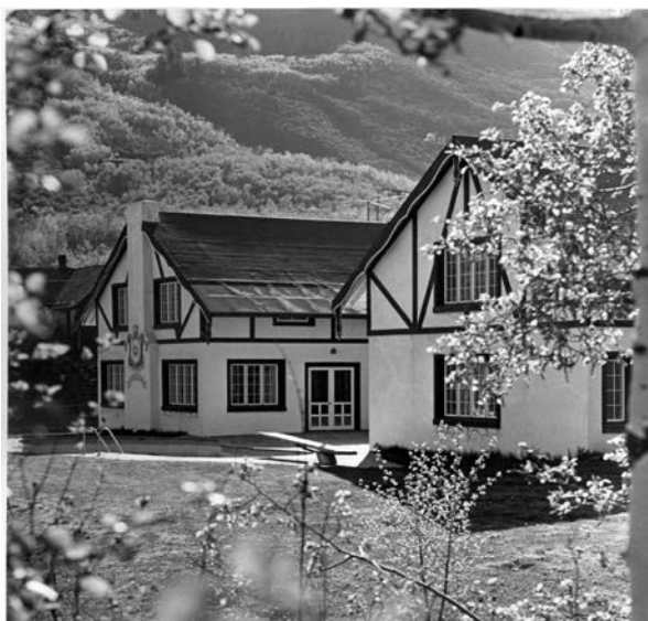
Cresta Haus, East Cooper Avenue, since altered
